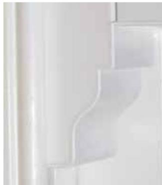
*3. Continuous Sash Horn Detail*
